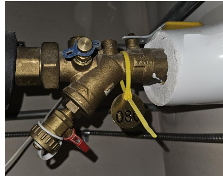
Typical strainer – clean out twice per year
